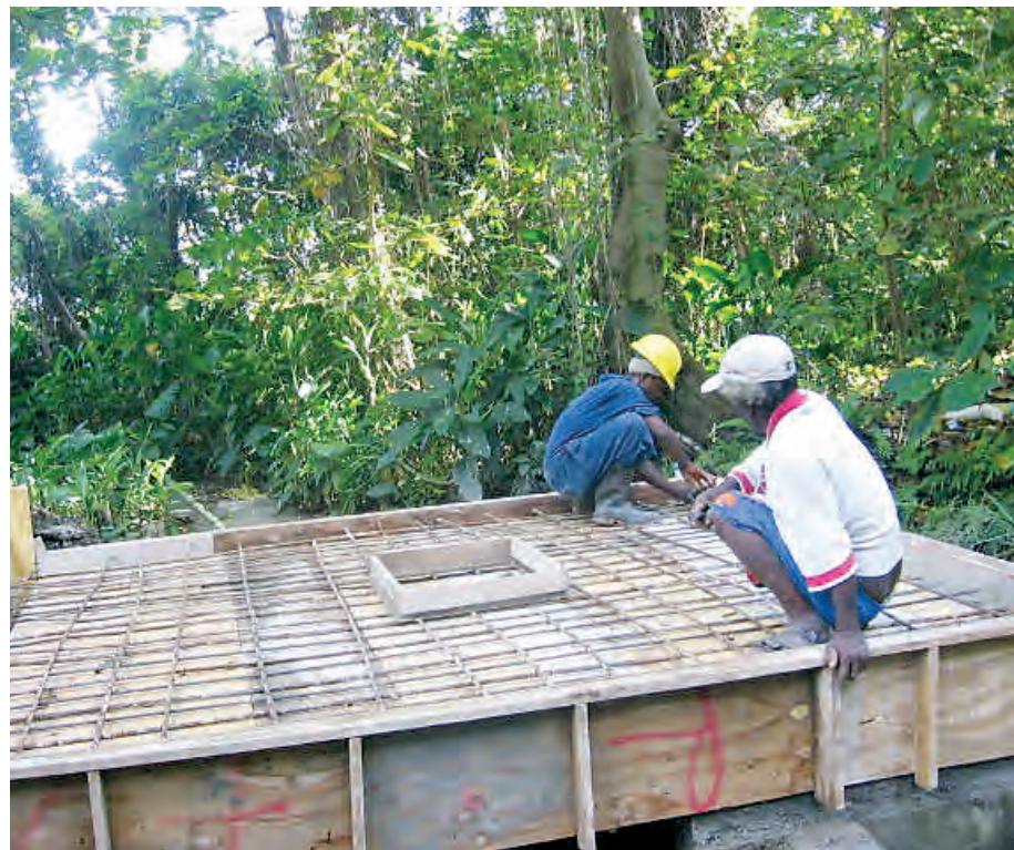
Workmen building check dam at Roselle in St. Thomas
