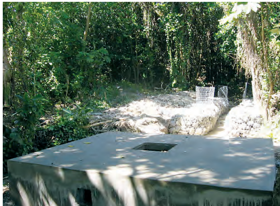
Completed check dam
