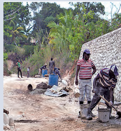
Road rehabilitation work
