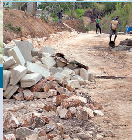
Tyre barriers and road rehabilitation work
