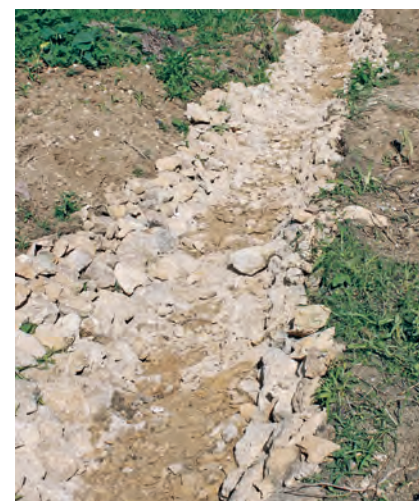
Stone layered drain
