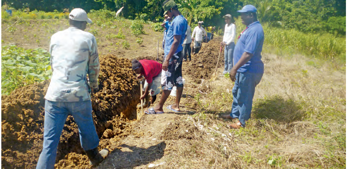
Above: Head drain construction Below: Pineapple/trash barrier and mulching
