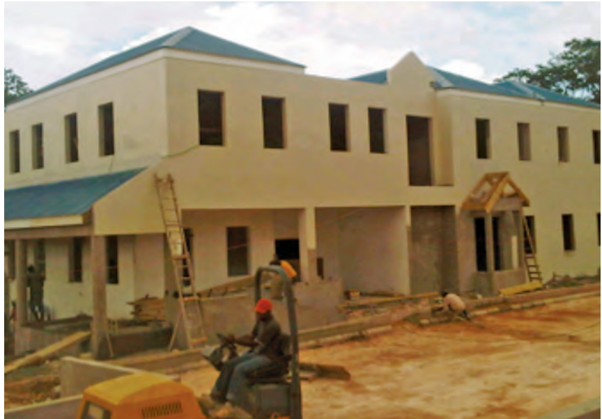
Trelawny parish office under construction.
