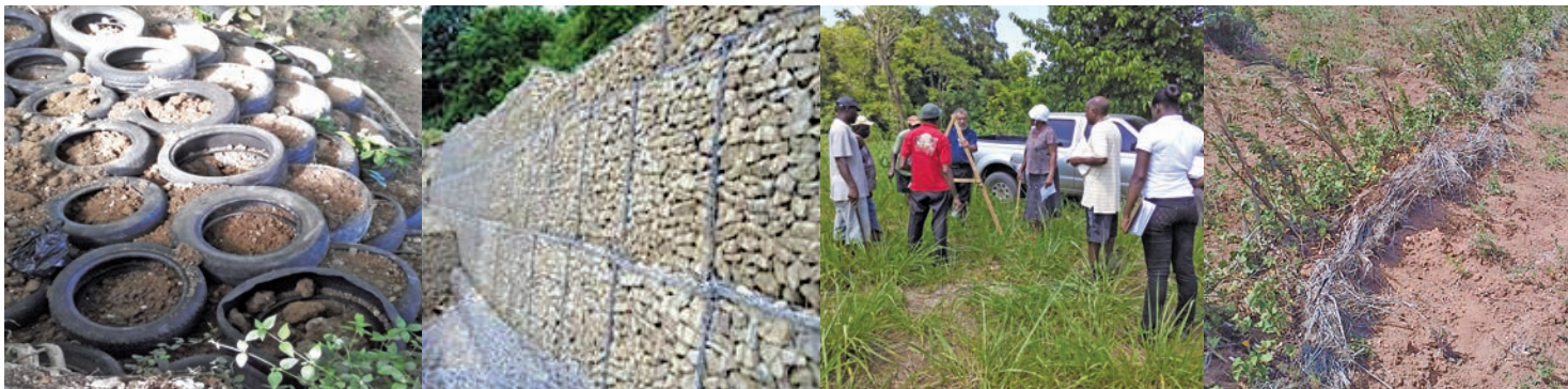
Land Husbandry Activities Check dam from recycled tyres, retaining walls using gabian basket, demonstration showing the use of the A-frame and mitigating soil erosion with trash barriers.
