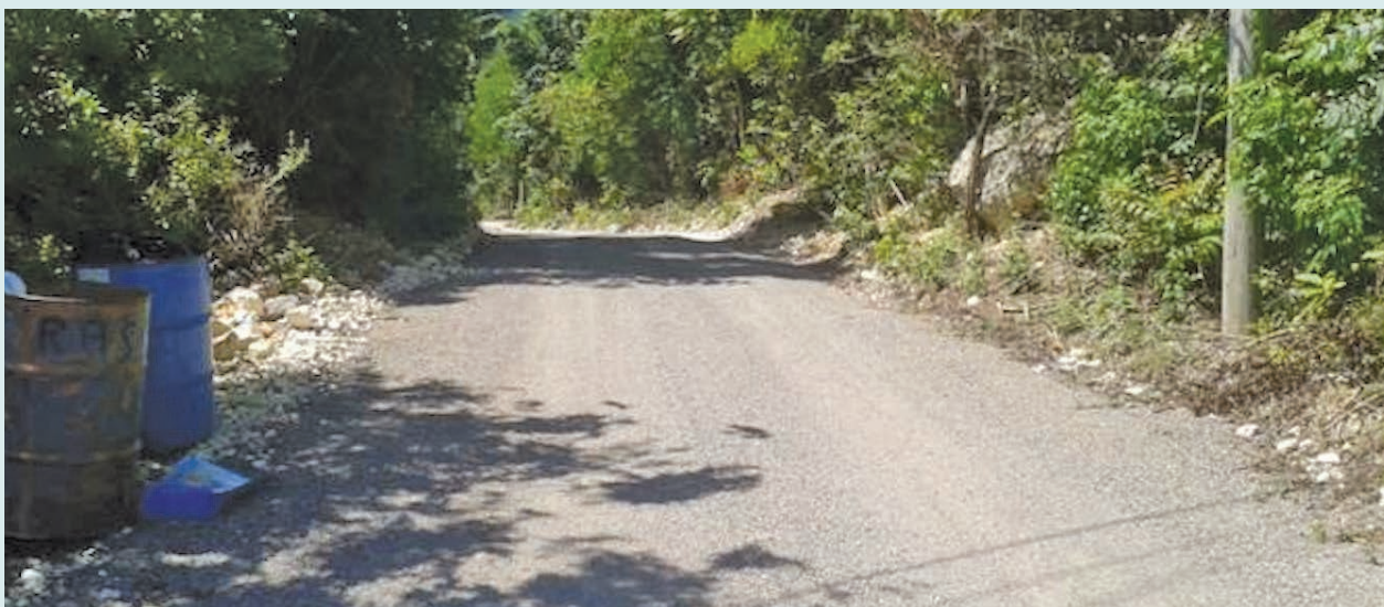
Section of a rehabilitated road
