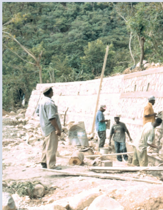
Retaining walls under construction.
